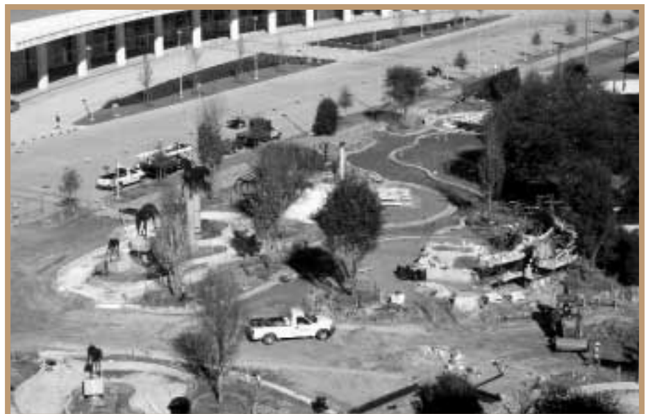
Rodeo attendees could look down on the Plaza’s construction from Reliant Stadium during the 2003 Show but will be able to stroll through and relax in the park-like setting for years to come.
