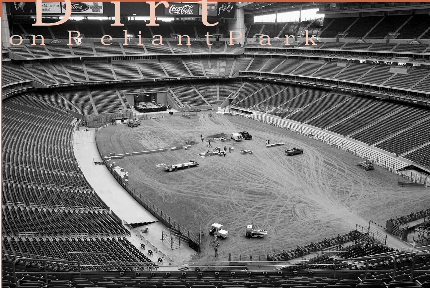
Before the broncs or bulls ever set hoof in Reliant Stadium, the portable grass field had to be removed and a dirt base created.
